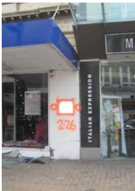
Figure 8 (International Team): Example of foreign date format. The size and location of the date is also non-compliant. Zero fields for victim information are also applied. Photo by Stuart Fraser.
