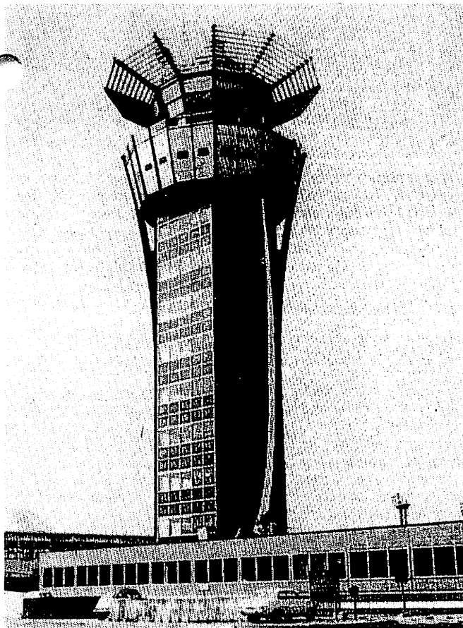
Evacuation of Tower Personnel using Otis System
